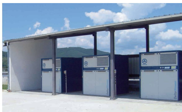
Blower station for air supply of the biological process
