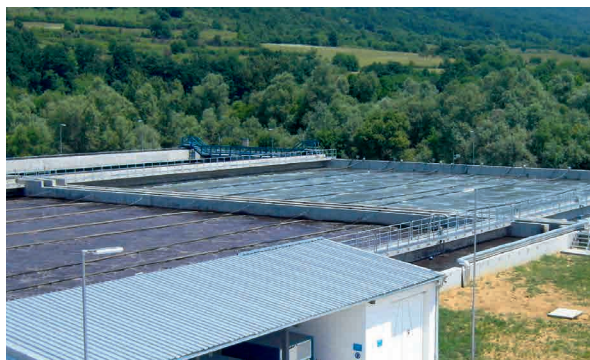
Bio-P zone, activated sludge basin and clarifier
