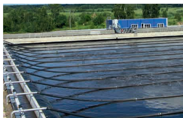
Integrated clarifier and activated sludge basin
