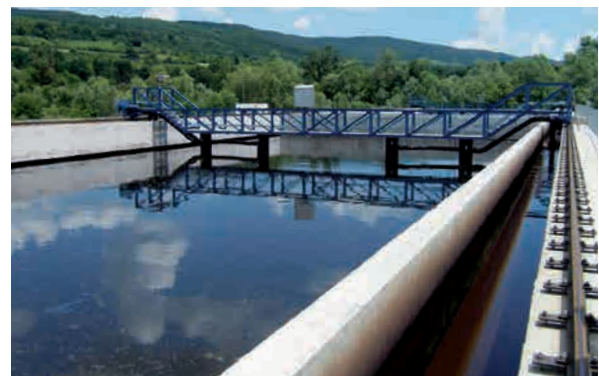
integrated clarifier and blower station
