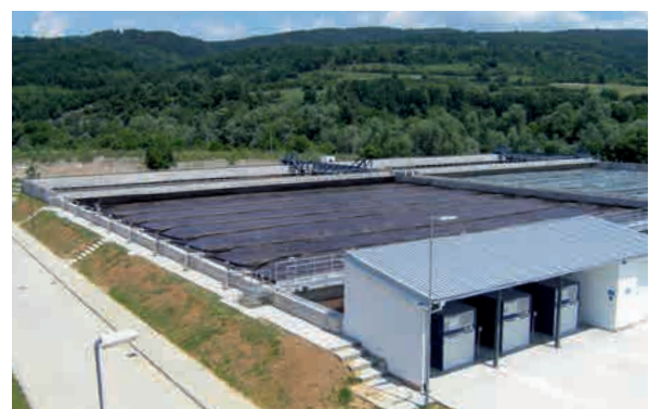
integrated clarifier and blower station
