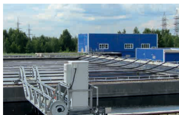
Integrated clarifier and activated sludge basin
