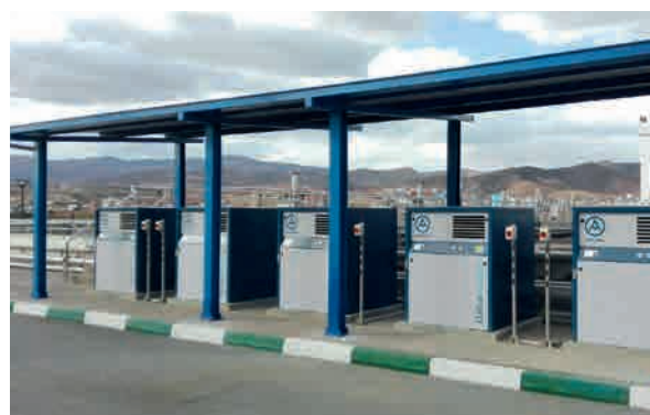
Compact station for mechanical pre-treatment, blower station
