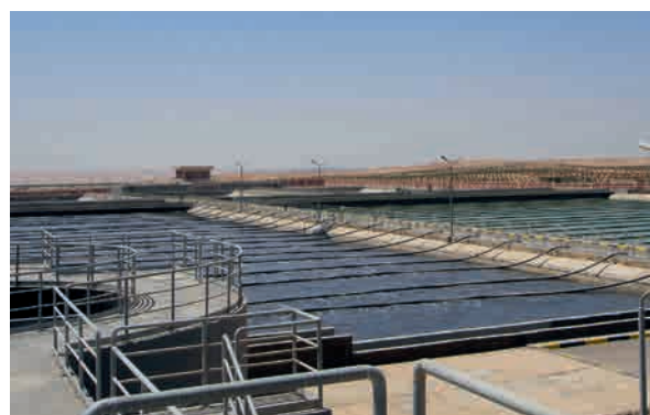
Sand removal facilities and activated sludge basins
