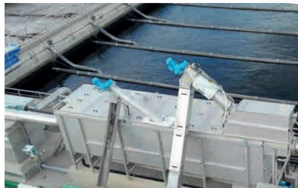
Compact station for mechanical pre-treatment, blower station
