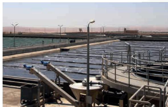
Sand removal facilities and activated sludge basins
